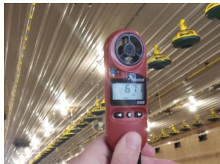
Their tunnel ventilation hit 671 feet per minute during a wind speed test.
