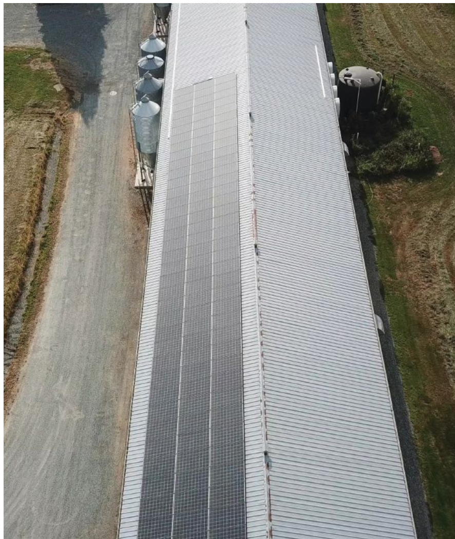
In 2016, Stewart Ritchie of S. J. Ritchie Research Farms installed solar power, rainwater capture and other energy-saving concepts in order to begin gathering more data on sustainability.
