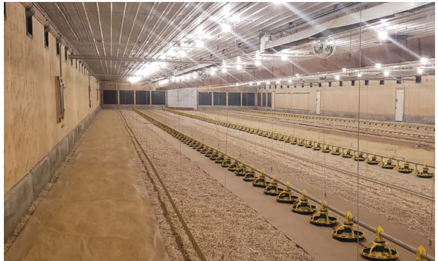
All feeding, drinking and 15 54-inch fans per barn were supplied by VAL-CO.
