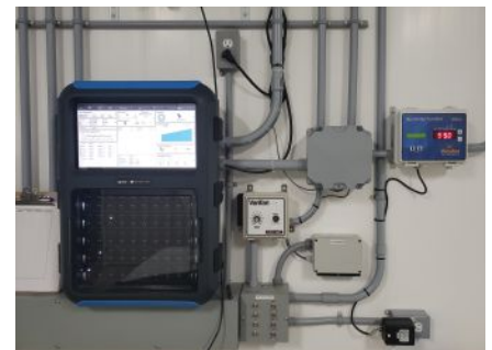
Each barn includes a Rotem Controller, which the producers have found to be simple to use.
