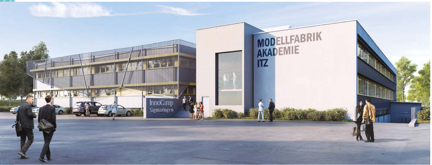
The InnoCamp Sigmaringen, where research projects on sustainable packaging concepts are being carried out in the near future. (architektenwerkgemeinschaft weinbrenner.single.arabzadeh)
