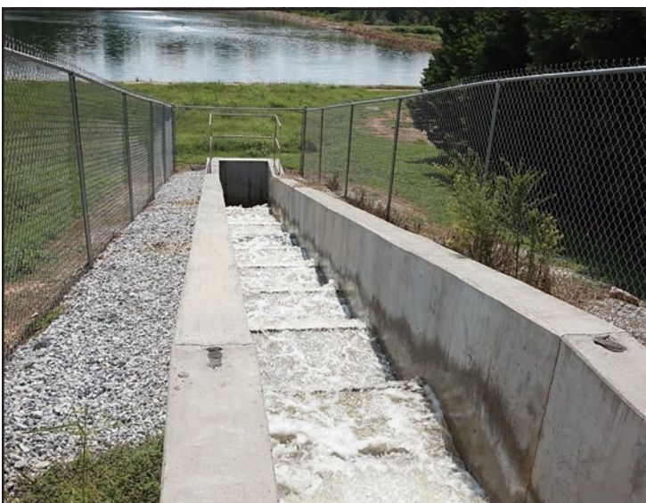
Cascading aeration transporting ultra-filtered and UV-disinfected treated wastewater to discharge. John Pierson
